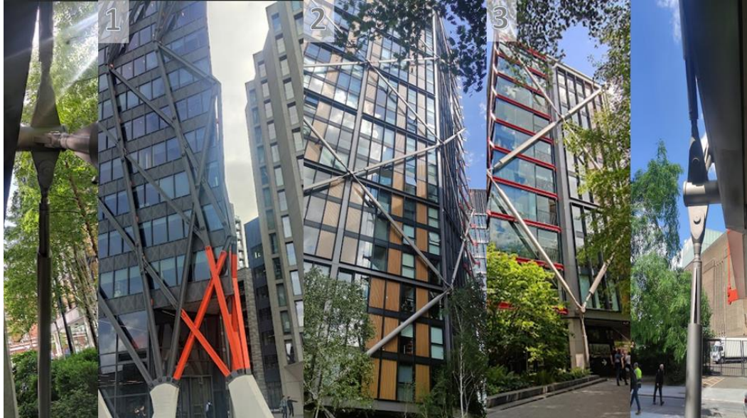
Fig. 7. Steel bracing (source: own study Daria Jasińska (photo taken in June 2023))
